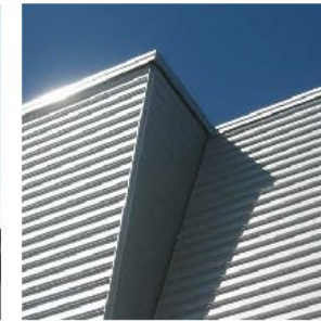
Trapezoidal Metal Cladding- Light and Dark Grey
